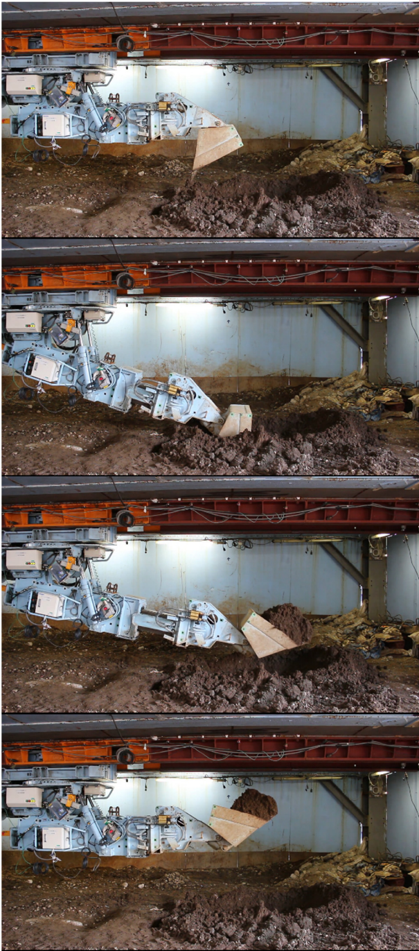
Fig. 8 Soil mountain removal by the PD control
